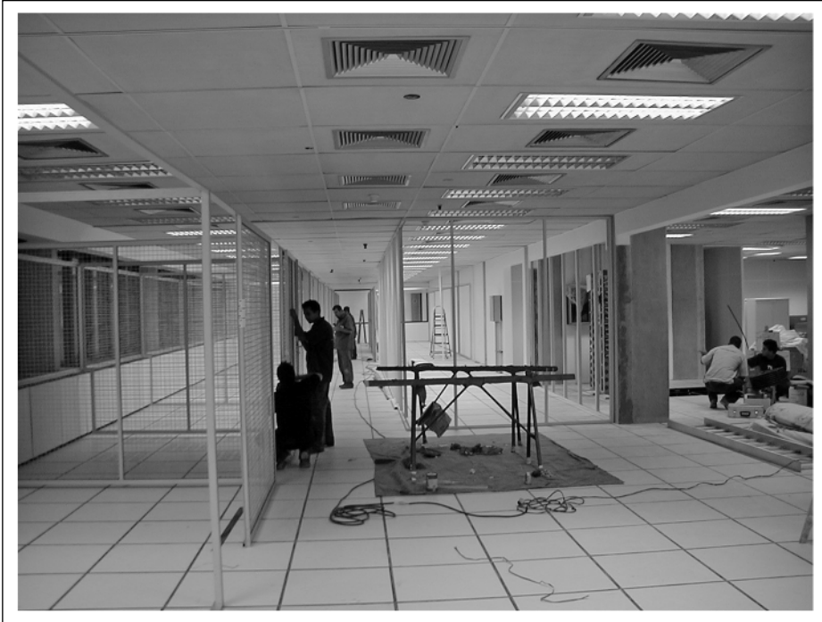
Figure 5-4 Laying fixtures and cables for data-center PODs.
